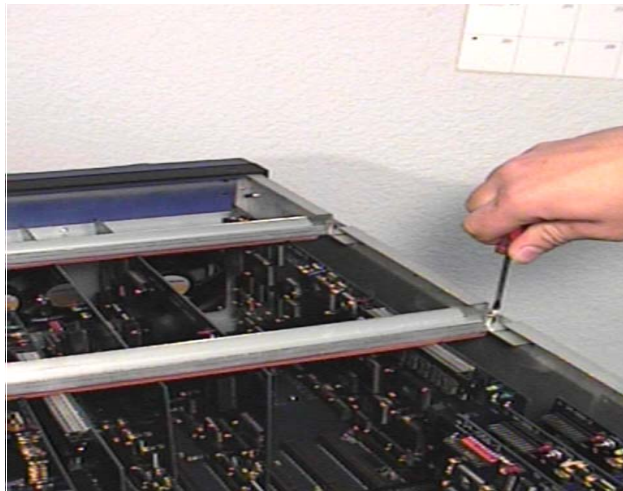
Figure 1.3: Removal of Retaining Bar
